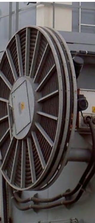
Double Monospiral Spool , with two identical cables with large cross-sections.
